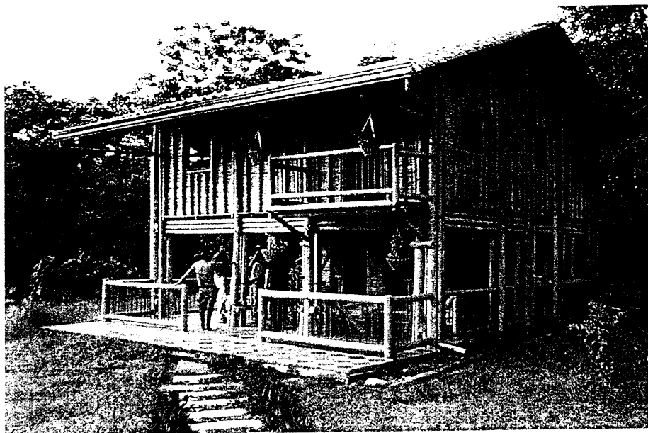
Figure 2. A house at the "Experimental Centre for Bamboo Construction". Other new bamboo structures also performed well during this earthquake
